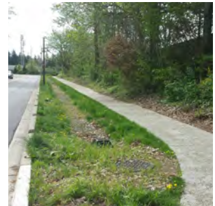
Example of curb cuts and porous concrete stormwater retrofit on 233rd Avenue NE
