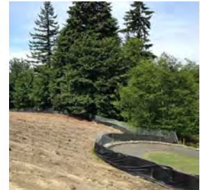
Erosion control features to prevent water quality issues during construction of the Sammamish Community and Aquatic Center
