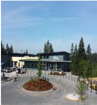
Sammamish Community and Aquatic Center green roof
