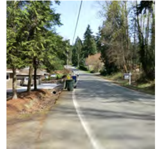
Example of ditch and culvert stormwater conveyance in Sammamish
