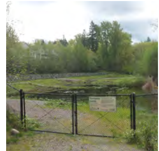
SE 8th Street stormwater pond
