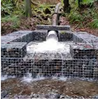
Evans Creek HDPE pipe outfall energy dissipation
