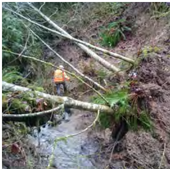
Landslide adjacent to George Davis Creek
