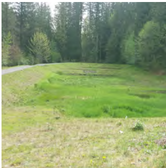
244th Avenue NE stormwater facility
