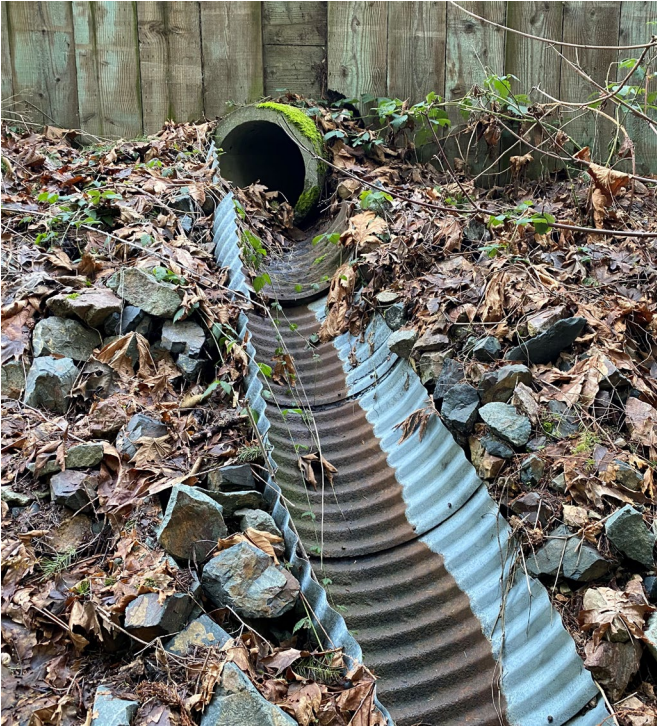
Photograph 9. Culvert 2 outfall with splash pad at station 40+50.
