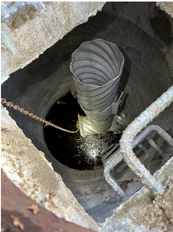
Photograph 3. Riser structure downstream of the existing detention pond at station 15+00.
