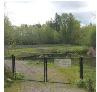
SE 8th Street stormwater pond
