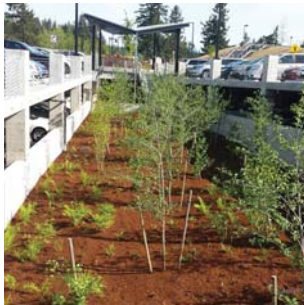
Stormwater detention vault at Sammamish Community and Aquatic Center
