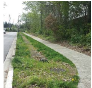
Example of curb cuts and porous concrete stormwater retrofit on 233rd Avenue NE
