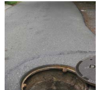
Manhole with cover removed
