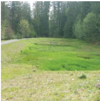
244th Avenue NE stormwater facility
