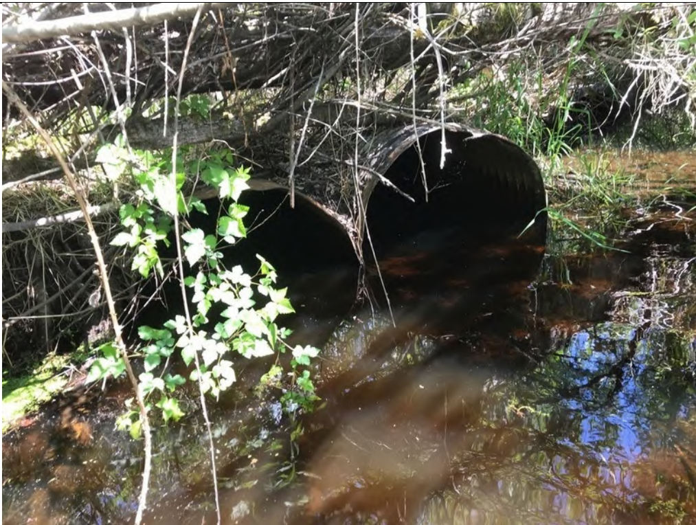
Photo 12. View of downstream side of culverts under SE 42 nd Street.
