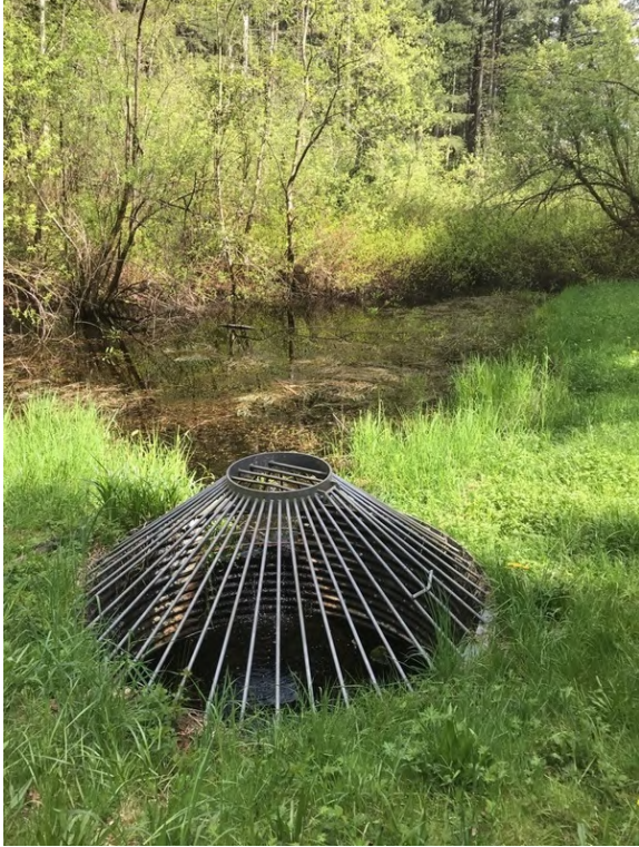
Photo 19. An eight-foot-diameter standpipe with a debris rack (birds nest) controls the flow of water from Queens Bog west into the upper reaches of the stream.
