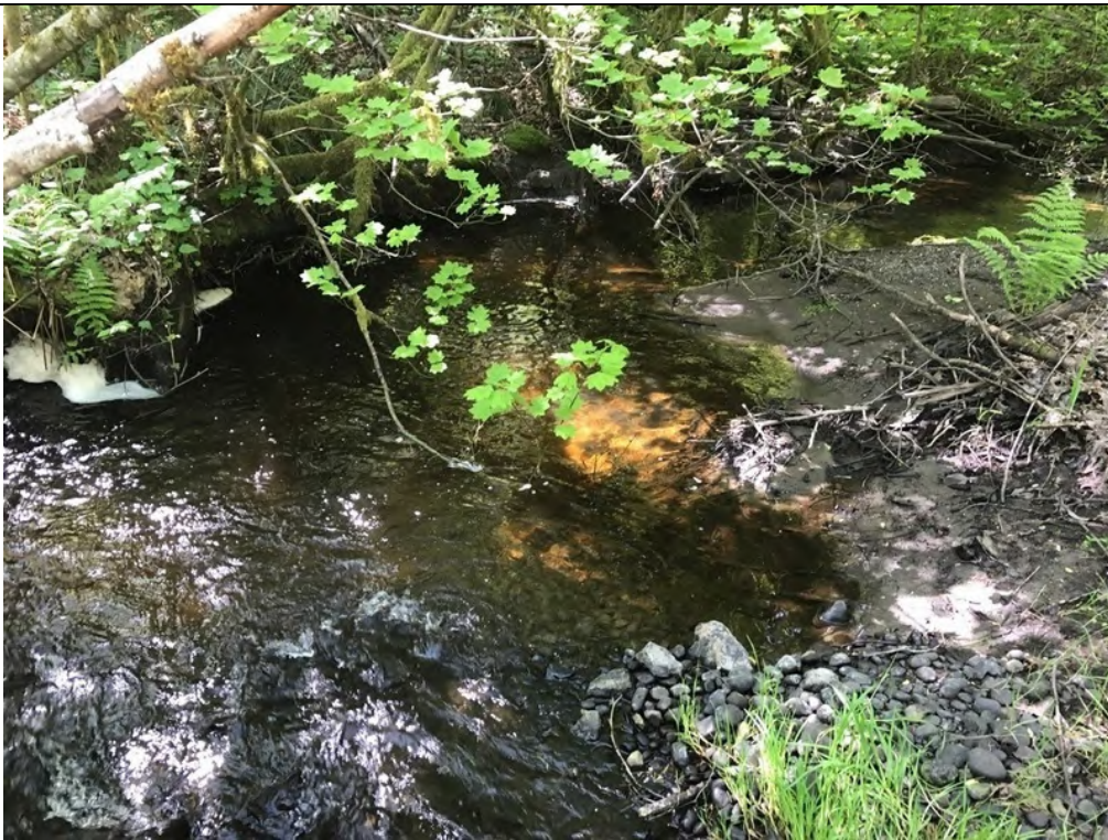
Photo 16. Laughing Jacobs Creek downstream of 230 th Way SE culvert.
