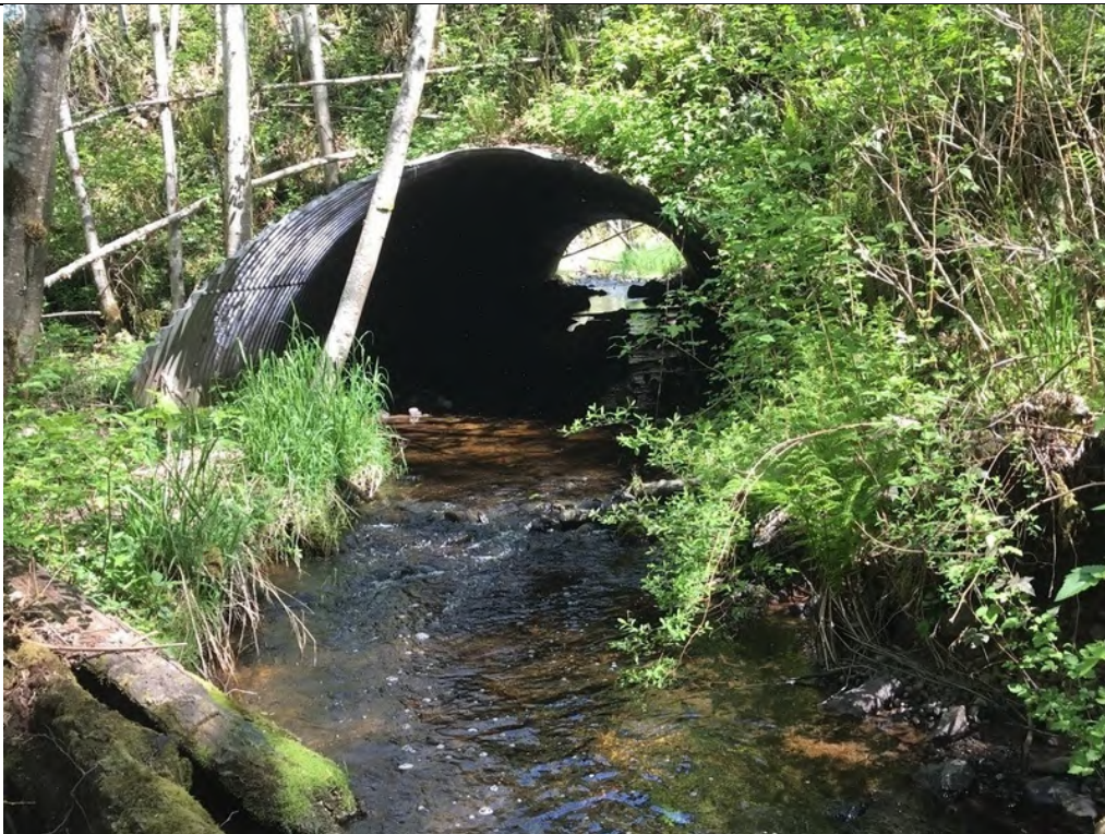
Photo 14. 230 th Way SE culvert crossing, looking upstream.
