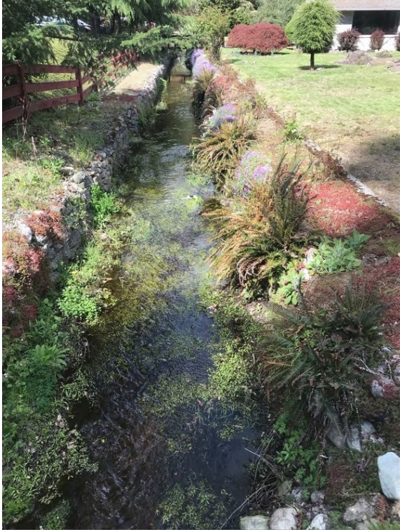
Photo 7. Immediately upstream of the Issaquah-Pine Lake Road SE culvert, the creek is channelized and has armored banks between a residence and the Lakeside Montessori School.
