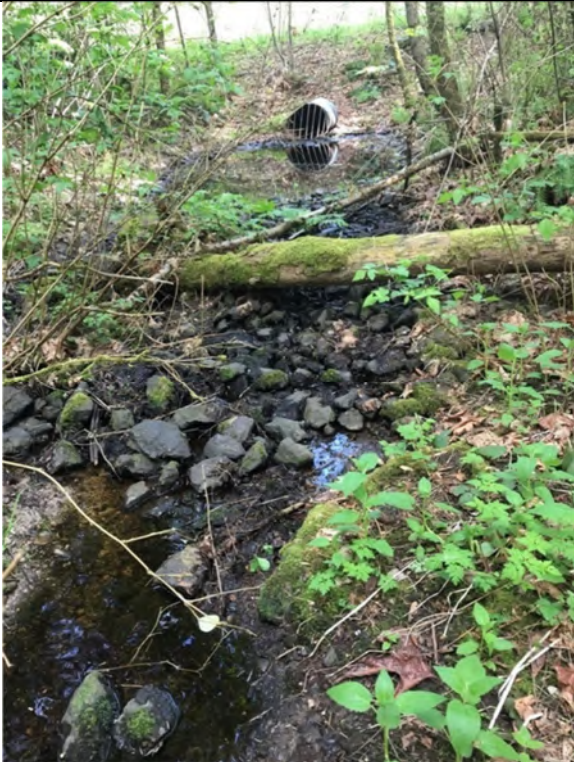
Photo 20. Headwaters of East Tributary at Klahanie Park wetlands; trail crossing is a fish passage barrier.
