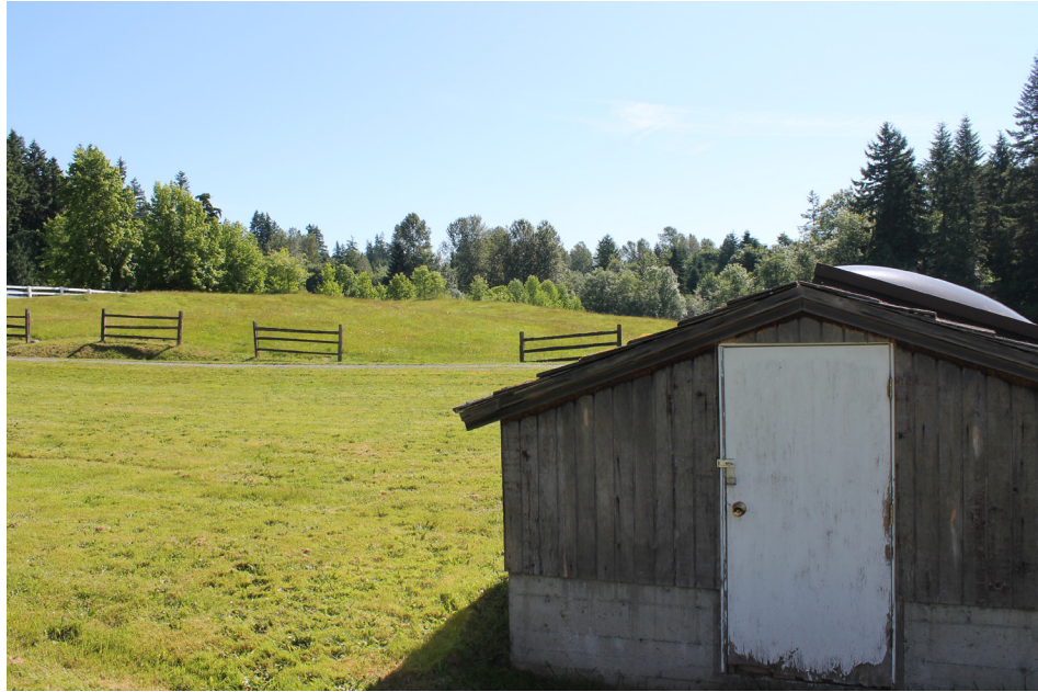
Well House, Site A
