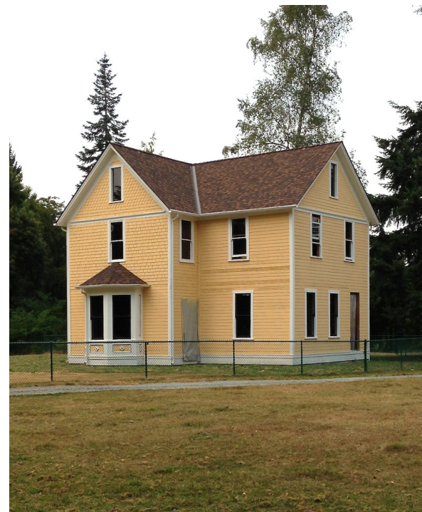
The Reard-Freed House, Site B
