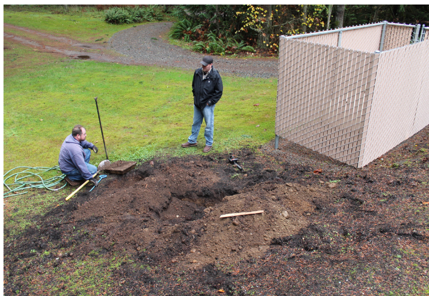
Existing Septic System Assessment, Site A
