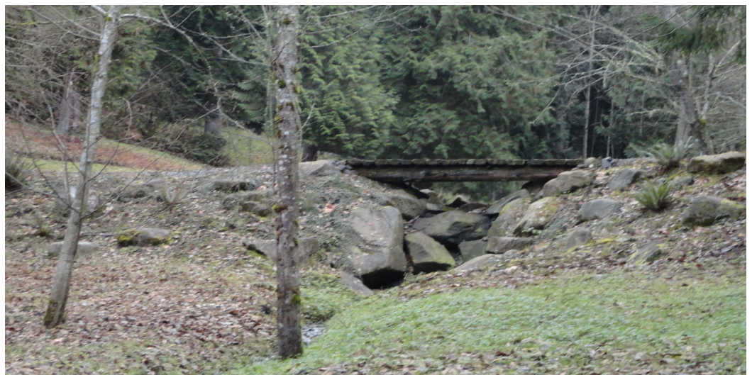
Stream Crossing, Site B
