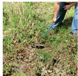
Roadside ditch in need of maintenance. Vegetation is blocking inlet to pipe.
