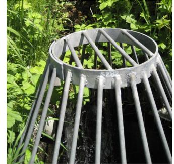
Example birdcage structure used to prevent large debris from getting into and clogging stormwater pipes. City crews inspect and maintain these facilities
