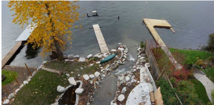
A reconstructed stream channel and shoreline restore habitat to the mouth of George Davis Creek—Kokanee salmon now spawn at the restored site (credit: The Watershed Company)
