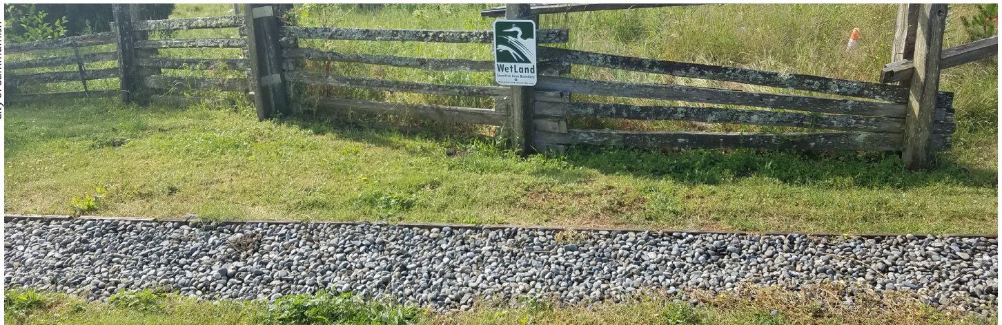
Dispersion trench to a wetland at the Sammamish Commons.
