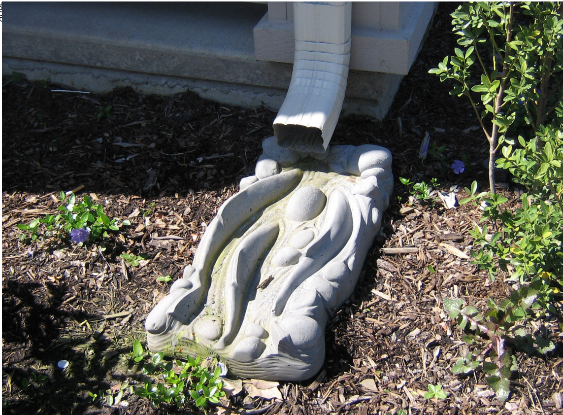
Example of a splashblock used to disperse stormwater runoff from a downspout.
