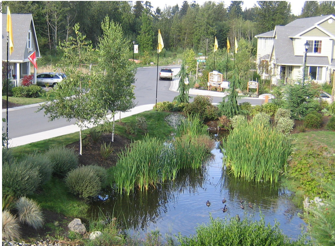
Example of a ground surface depression used to infiltrate stormwater runoff.
