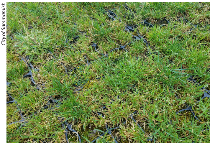
Example of a grasscrete (grassed modular grid pavement) parking area.
