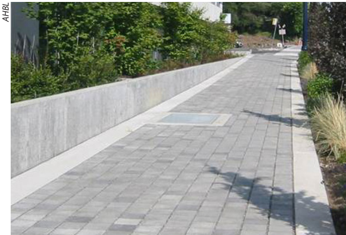
Example of a permeable paver sidewalk.
