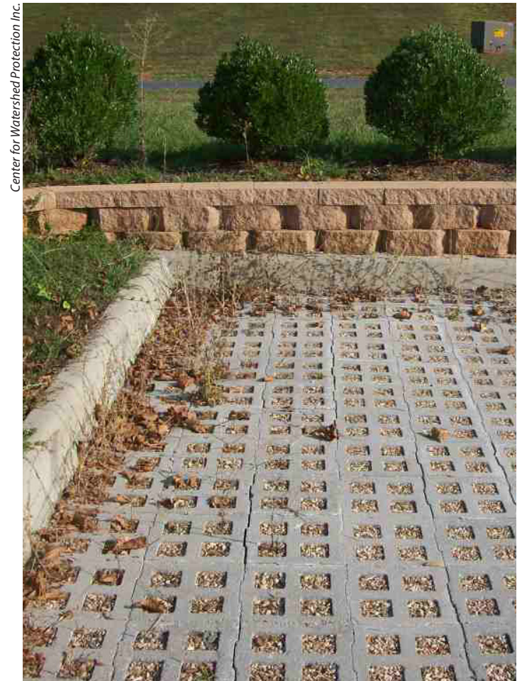
Example of a modular grid pavement parking area in need of maintenance. Leaves and debris pose clogging hazards, and reduce infiltration.
